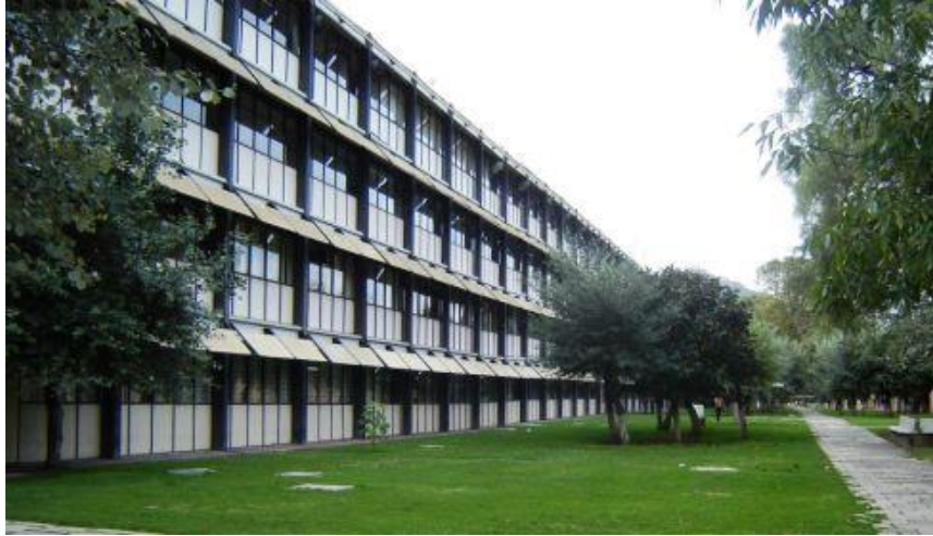
Fig. 2. Classroom, laboratory, library, auditorium and office buildings, and offices with linear steel structure.
